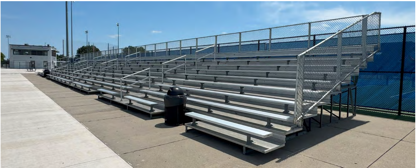
Image of the Existing Bleachers at North High School
